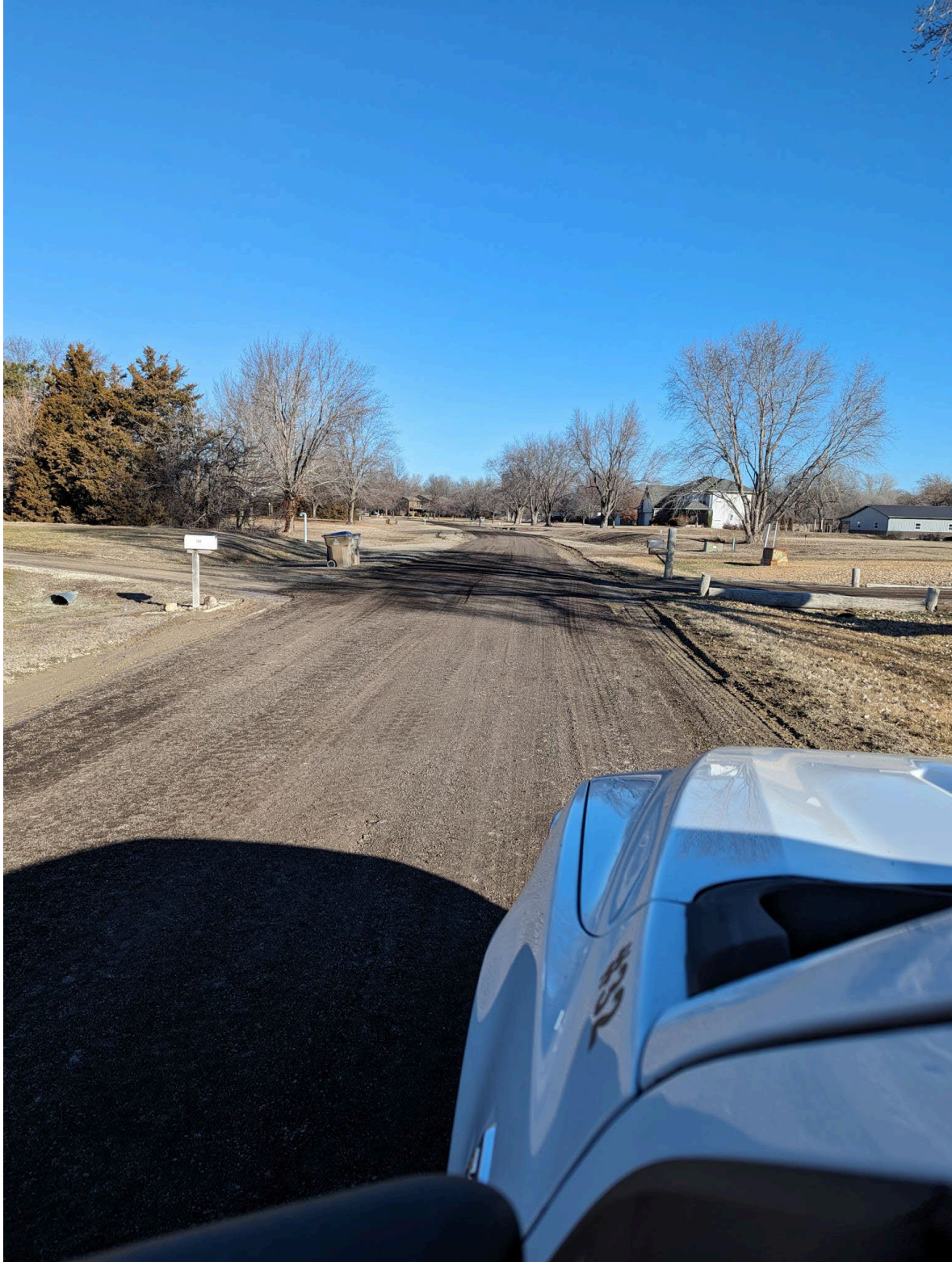
Chaparral with a new layer of asphalt millings. Staff was still packing the road when this picture was taken. This is our plan for Kessler also.
